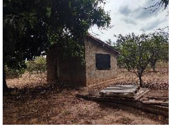
Agrochemicals Storage (Cooperative C)
